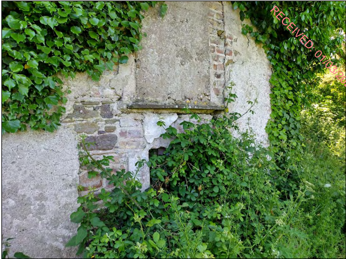
Plate 9. Small square-shaped building showing stone construction, external render, ground floor doorway and first floor window with a brick surround (blocked up).
