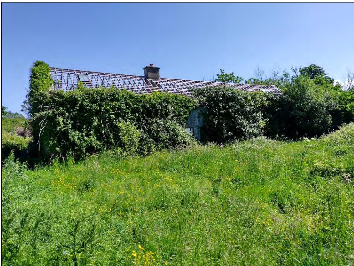
Plate 6. Single storey cottage representing the northern range of buildings depicted on the historic mapping. Slate roof has been removed and is overgrown with ivy.
